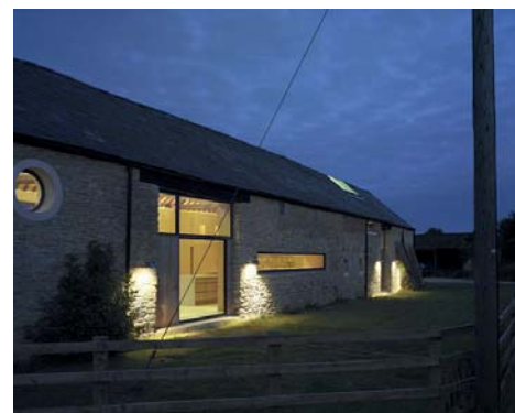
Nye store vinduesåbninger i facaden Pinions Barn, Simon Conder Associates
