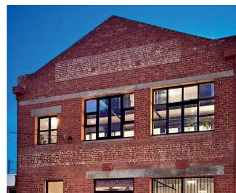
Nye store åbninger i facaden Abbotsford warehouse, ITN architects
